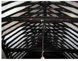
The roof in the **North chapel** is a miniature hammer-beam roof of three bays (below, right). It is the only example of its type in a Middlesex church.
